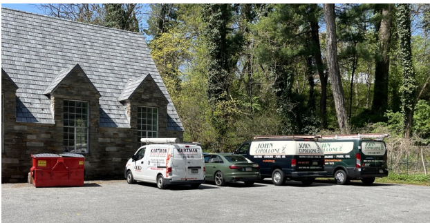
~Keeping on top of repairs around the building ~
